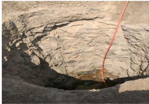
Fig 2. Dry dugwell, Inconsistent jointing pattern.
